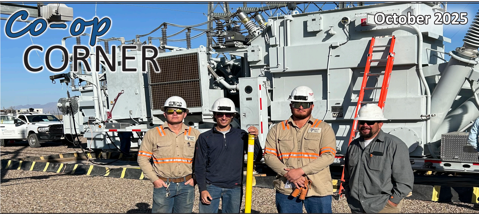
SEC Employees (L-R): Nik Landry, Norman Finley, Michael Trujillo, Zach Ortega pictured with Tri-State Mobile Substation
