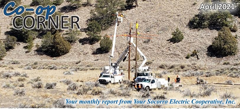
SEC linemen - Layne Bugayong, Mathew Dempsey, Glenn Calvert, Jason Otero, Mike Reiff and Colby Kerr, are replacing a 3-phase pole in Datil Canyon under engergized conditions providing uninterrupted power for our Members.
