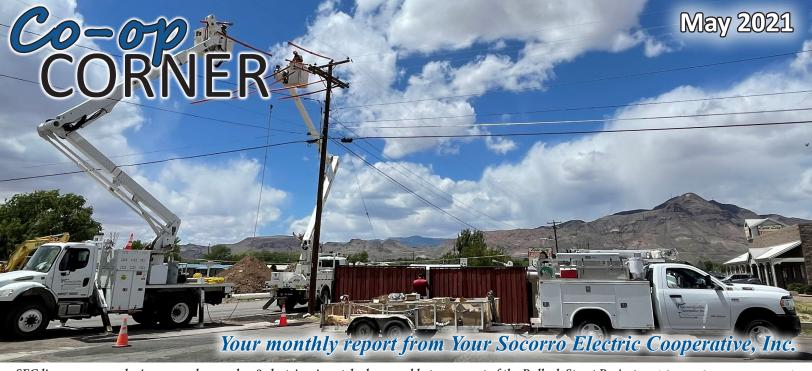
SEC linemen are replacing a very busy pole - 8 electric wires, telephone, cable tv - as part of the Bullock Street Project. (Photo credits - Rauni Montoya)
